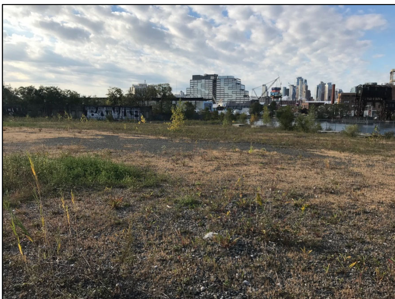
Photograph 6: Condition of Former Generating Station Building Foundation
