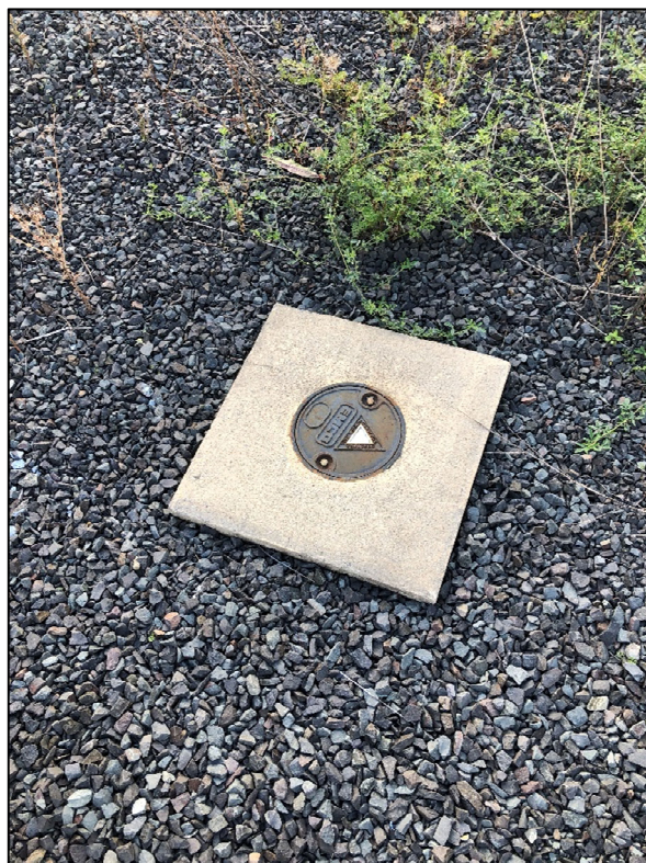
Photograph 2: Condition of flushmount monitoring well
