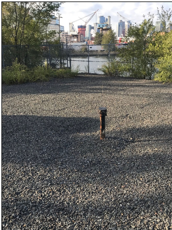
Photograph 1: Condition of stickup monitoring well in South Excavation Area with minor rutting
