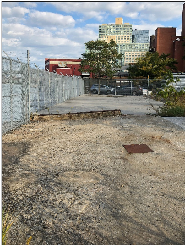
Photograph 4: Condition of Remnant Basement Slab
