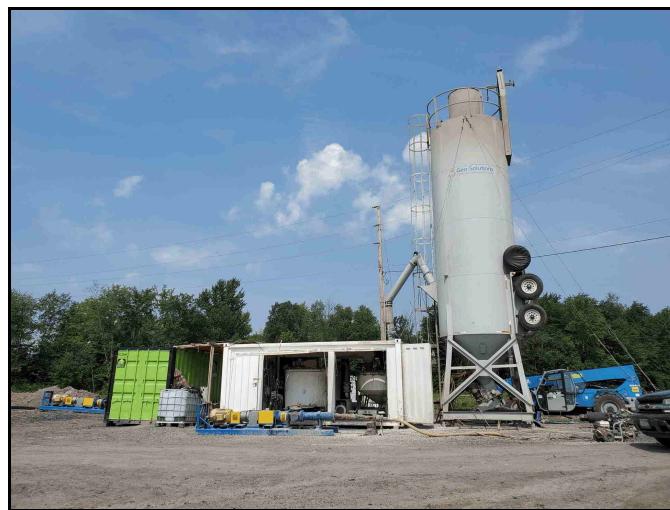
Construction equipment at Stage 5
