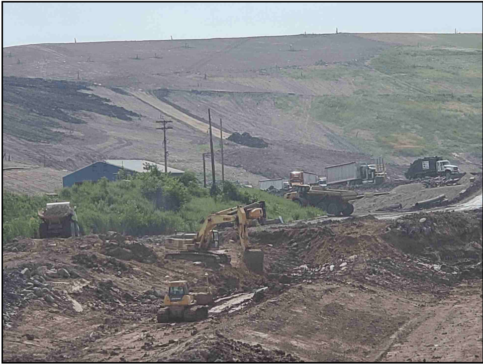
Soil excavation and construction at Stage 5
