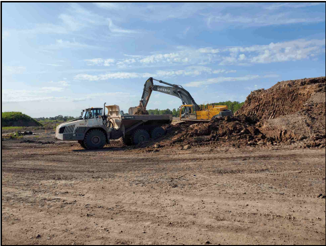
Loading of soil at Salcman Road materials storage area
