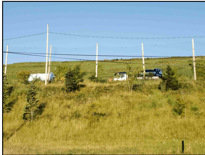
Leachate collection system maintenance
