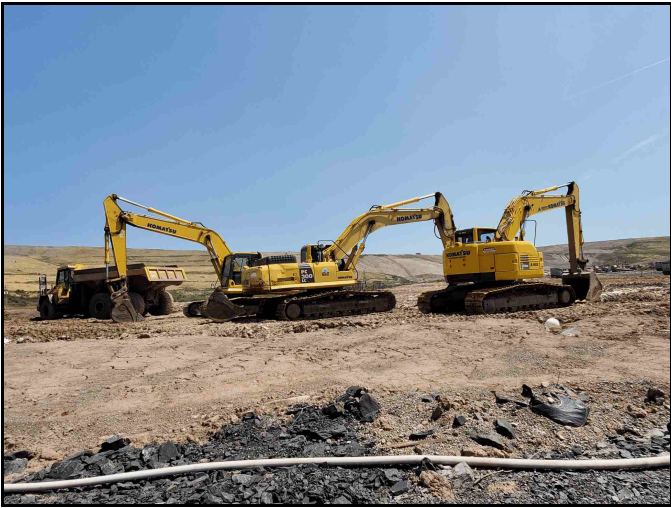
Construction activities and excavation equipment at Stages 5 and 6
