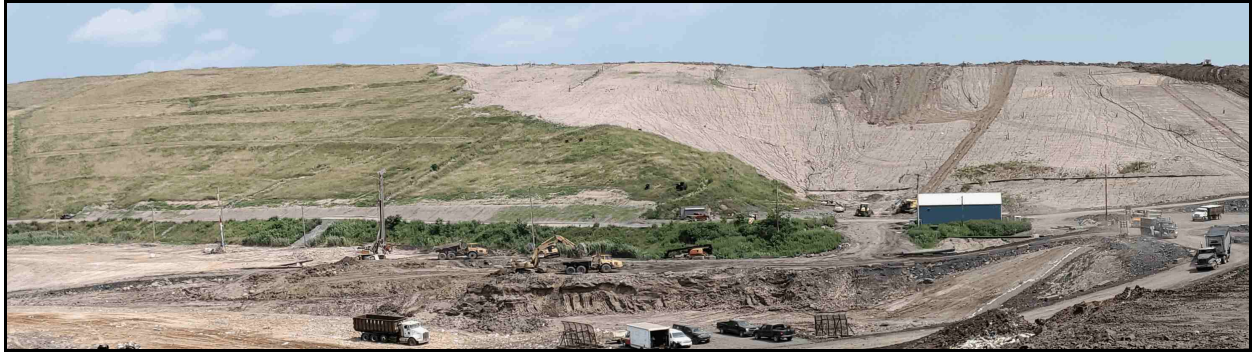
NEX soil unloading and placement, viewed from west
