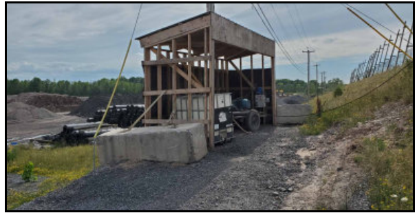
Odor neutralizing systems in noise enclosures
