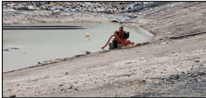
Dewatering pump adjacent to Stage 6
