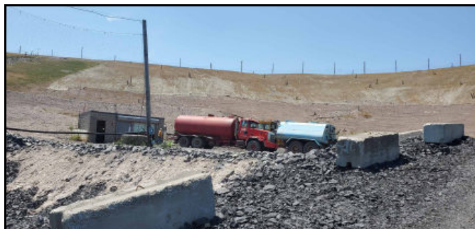
Leachate collection system cleaning at NEX
