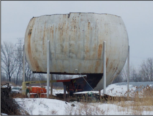
Demolition of the gas holder that was used to store excess coke oven gas prior to use in the coking process or being sold for off-site use (February 2021).
