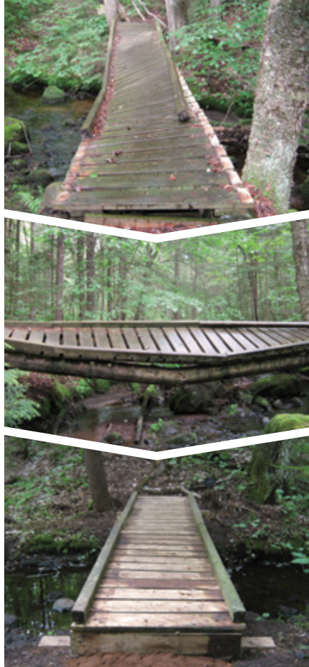
Above: SCA crews replaced the old bridge at 13 th Lake Inlet with a much sturdier one. Below: Saws and sweat are part of the experience. Crews stand on the Slim Pond Bridge, which they constructed using nearby timber resources and a cross cut saw.
