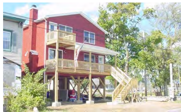
Figure 29. Home repaired to VE Zone standards, Stony Point, Rockland County, N.Y.
