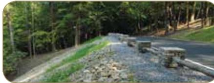
With EPF funding, a hillside and roadway used to access the Native American Council Grounds area of Letchworth State Park was reconstructed. The road collapsed in a 2011 landslide, closing off public access. The project included construction of historic Civilian Conservation Corps-era hand-laid stone piers and locust guiderails. Known as the "Grand Canyon of the East," with three major waterfalls as high as 600 feet, Letchworth receives about 650,000 visitors annually.
