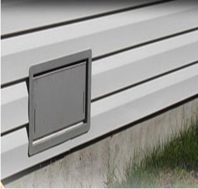
Figure 24. Engineered flood vent. The vent automatically opens under the pressure of water.
