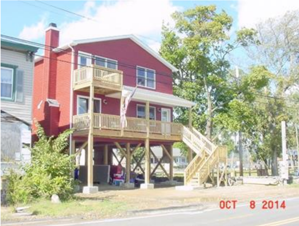
Figure 22. Home repaired to VE Zone standards, Stony Point, Rockland County, N.Y.
