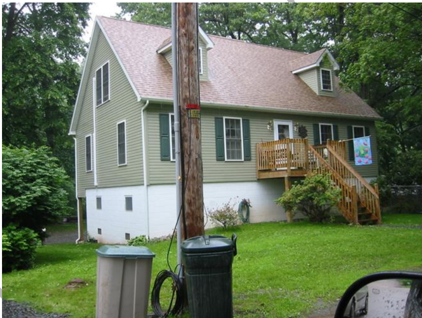
Figure 20. Example of properly elevated home with flood vents.
