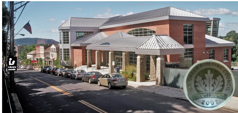
The village and town of Ossining, both Climate Smart Communities, serve residents with a new library, the state's first public building to meet the Leadership in Energy and Environmental Design (LEED) standard. (Photo courtesy of Amiaga Photo, Inc)
