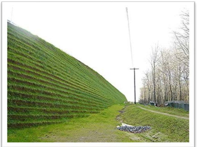
Examples of mechanically stabilized earth (MSE) berms similar to what will be used along the northern and northeastern perimeter of the Dunn facility.
