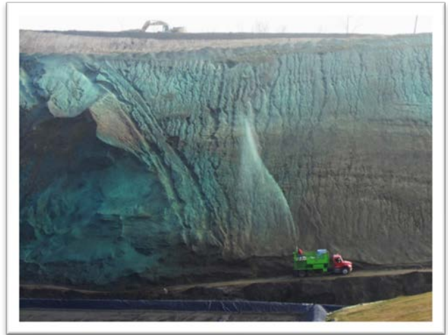
DEC requires hydroseeding at the Dunn facility to stabilize the sand, reducing offsite dust issues.
