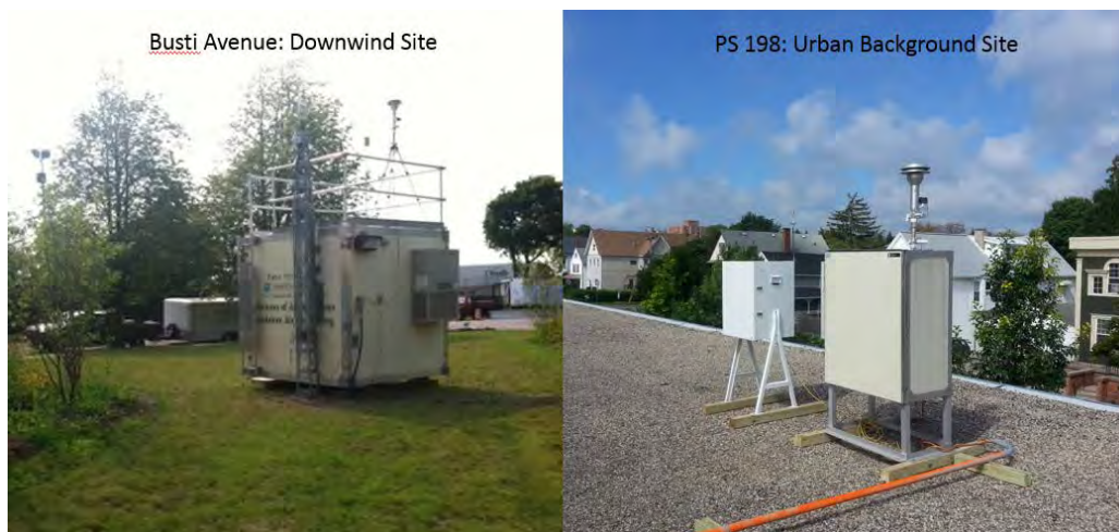
Figure 3. Study Monitoring Equipment
