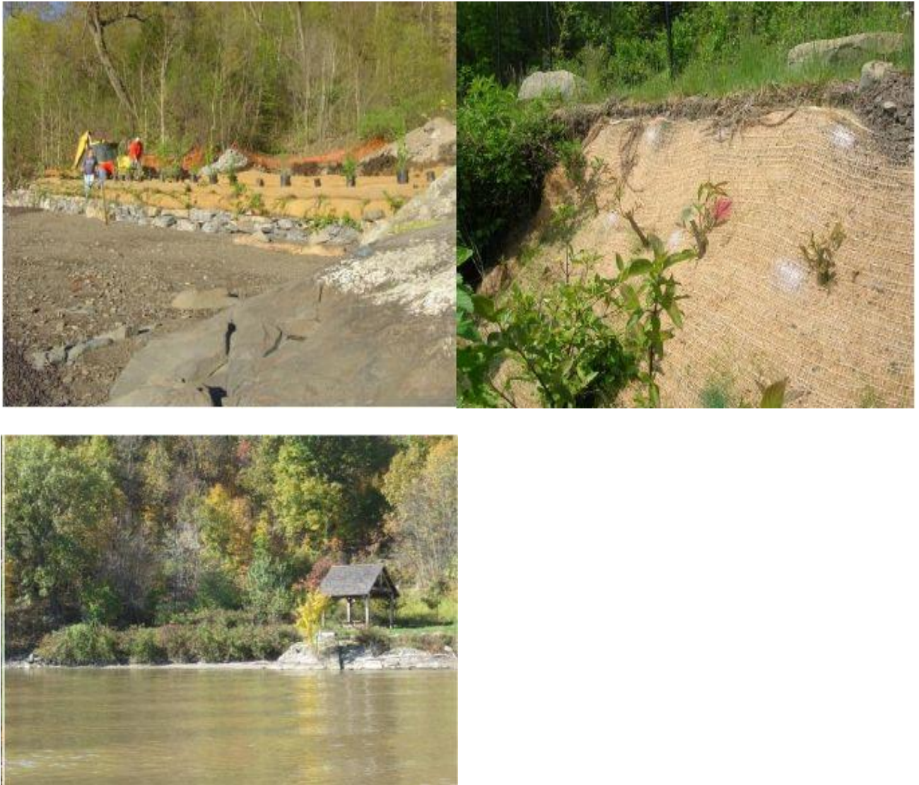
Figure 11. Example of stone toe protection with a vegetated slope using biodegradable geotextile and shrubs, upper left and right. Photo at left shows established shrubs and stone (toe at high tide), six years after installation at Esopus Meadows, NY. Photos courtesy of Creative Habitat Inc.
