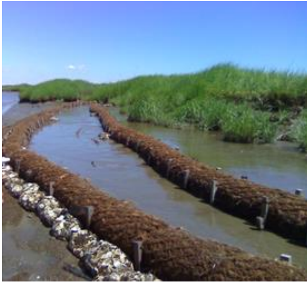
Figure 9. Fiber roll and bagged shell edging. Photo credit: Dave Bushek.
