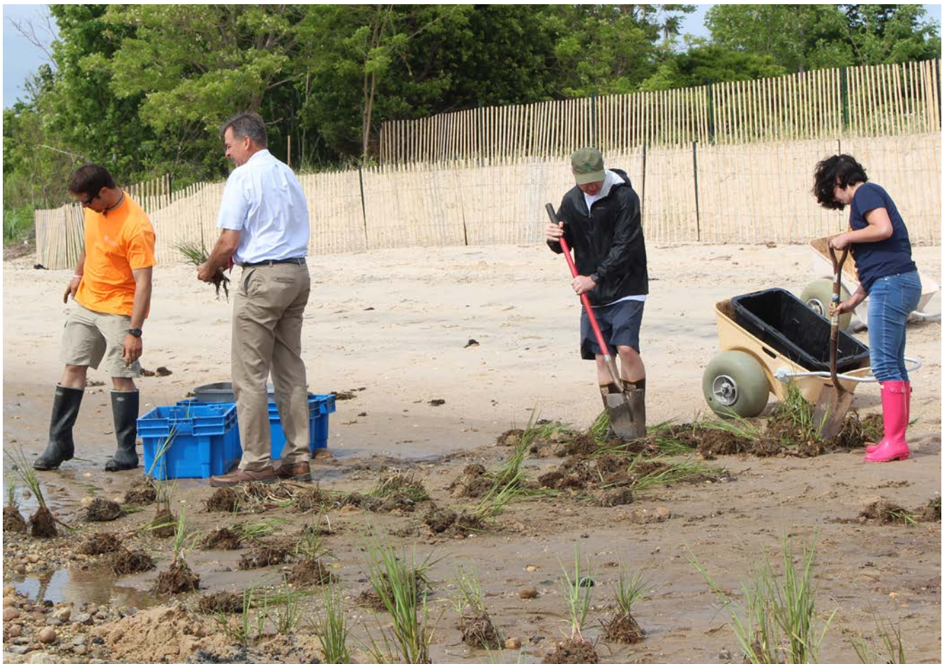
Students participate in installation of living shoreline at Widow's Hole Preserve.
