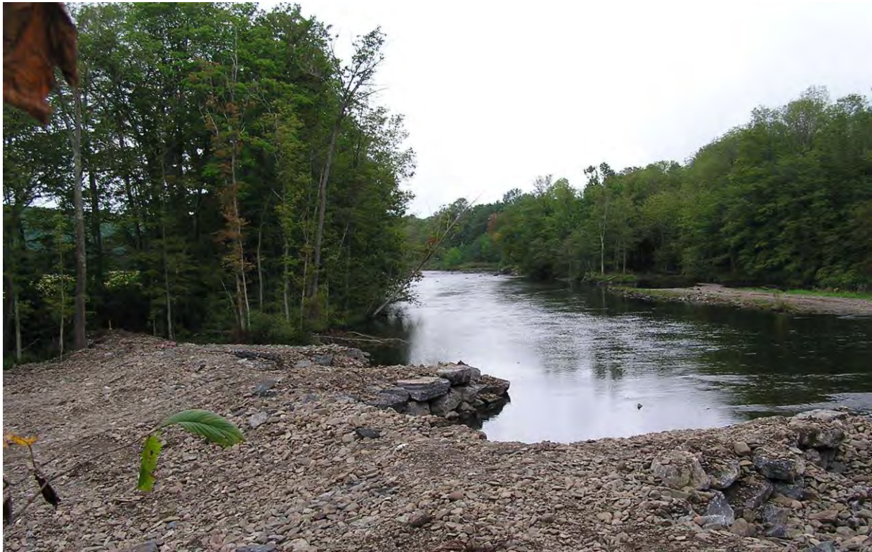
Figure 6. Bed sill structure across from the Salmon River Fish Hatchery. This structure blocked a secondary channel that was forming which would have diverted the main channel of the river around the mouth of Beaverdam Brook. The brook provides returning fish access to Salmon River Fish Hatchery.
