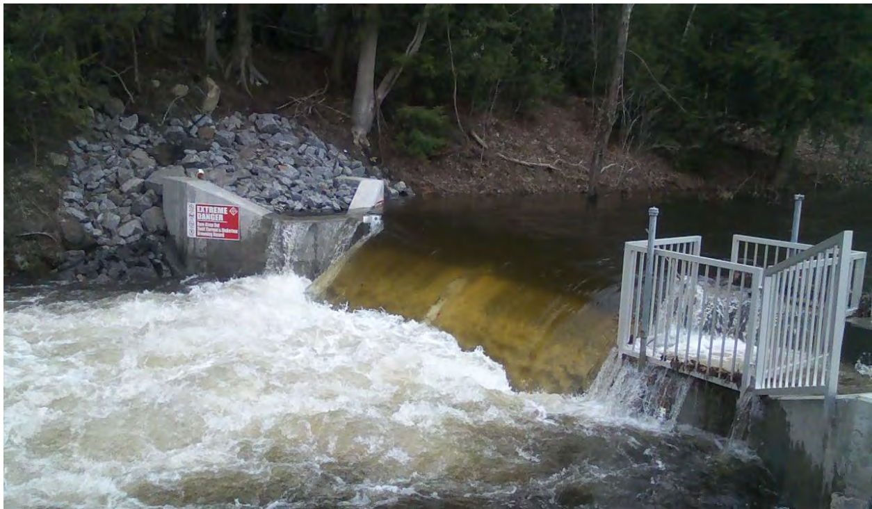
Figure 2. Sea lamprey barrier/trap on Orwell Brook. Stop logs are installed seasonally to exclude spawning sea lamprey migration and allow for fish passage. This alleviates the need to chemically treat for lamprey larvae above the structure.
