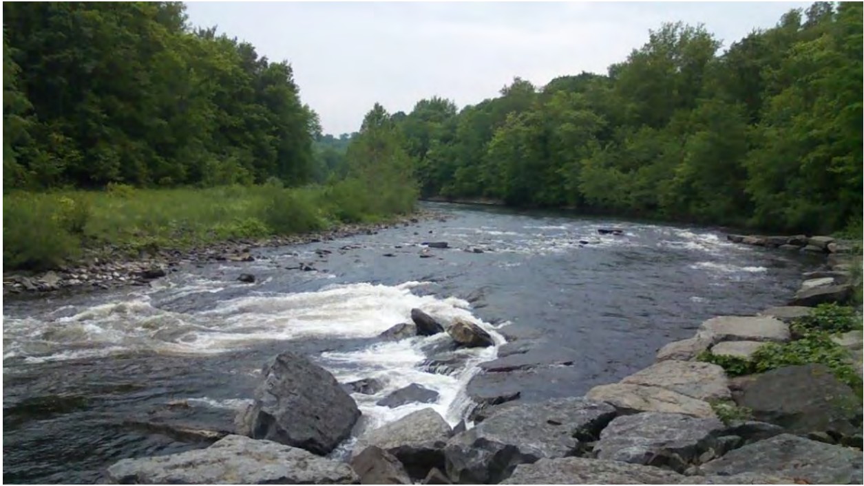
Figure 5. Restoration project in DEC's Upper Fly Fishing area consisting of a bankfull bench, vanes and a floodplain (opposite side of the river).
