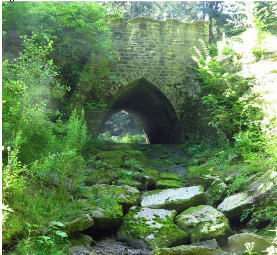
Figure 1. Stone road culvert on ASP Route #1.
