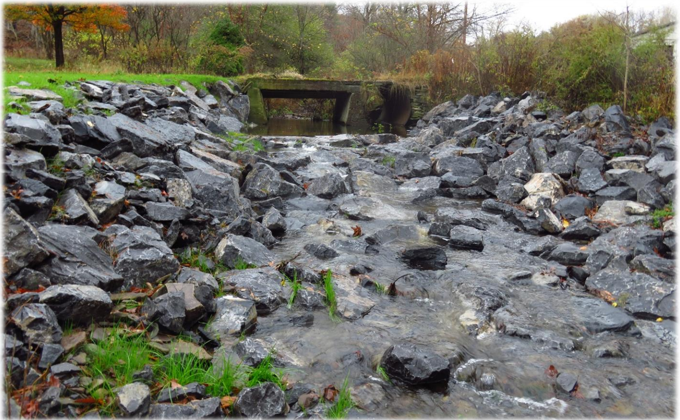
Figure 2. Culvert and engineered rock riffle on Indian Creek following project completion.
