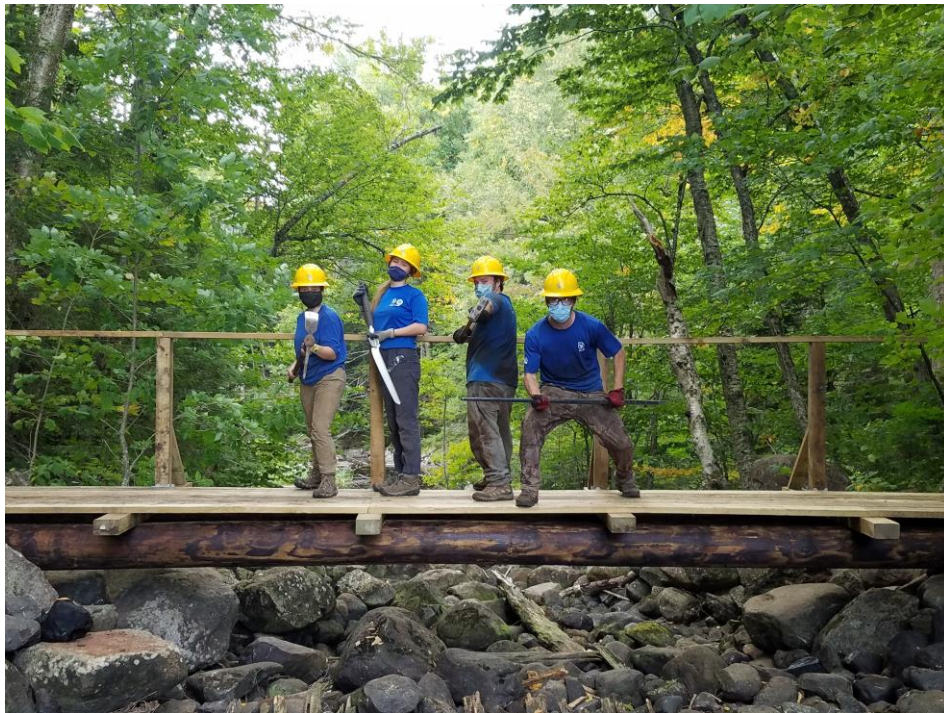
O'Neil Flow Bridge After
