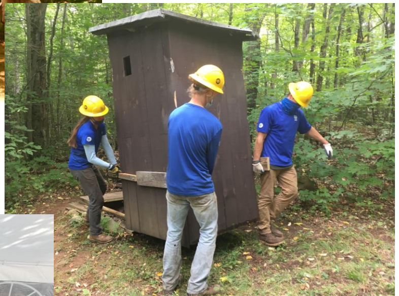
Relocating privies on Moose River Plains Road
