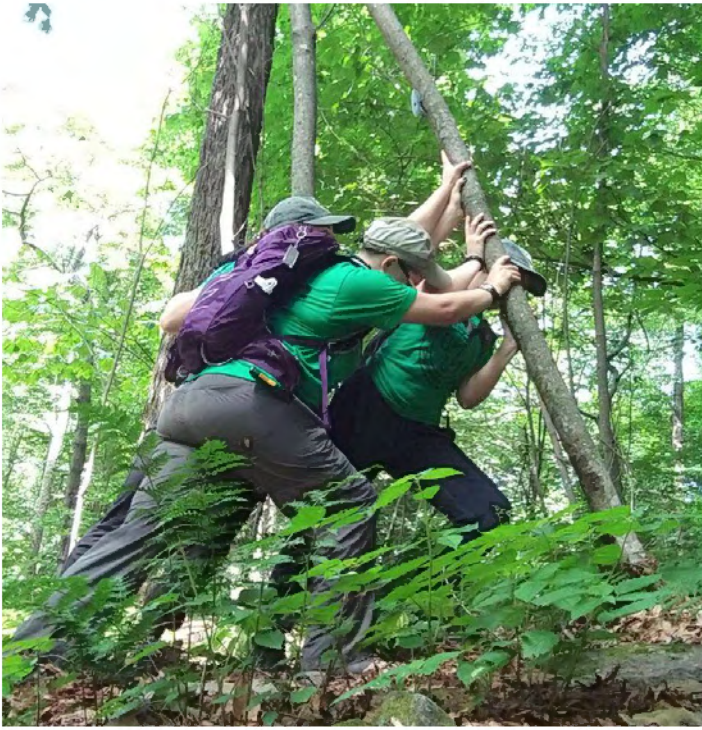
Removing blowdown from a trail, photo by Iona Hennessy
