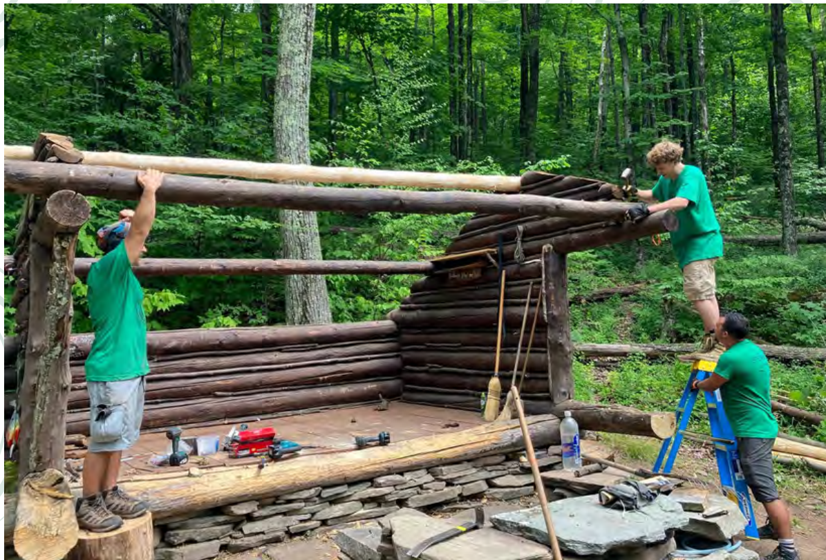
Josh, Liam, and Brandon attaching the front roof beam to the shelter
