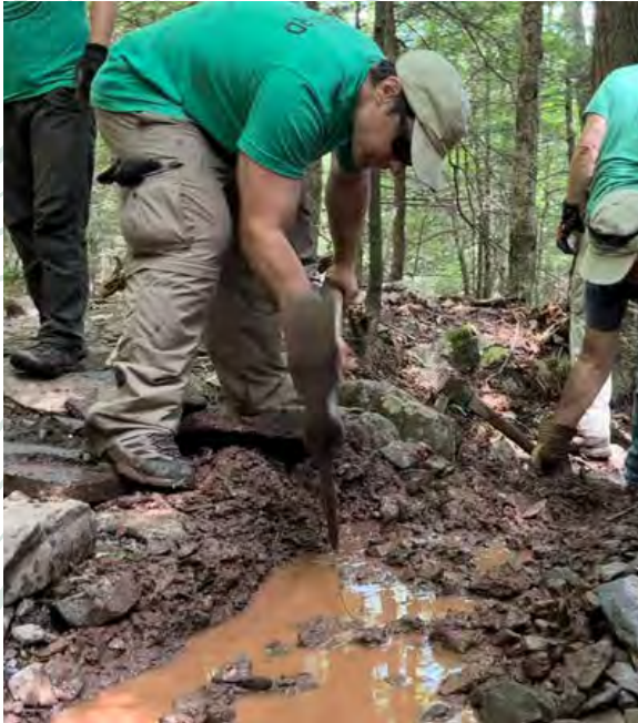
Digging out a drainage path to redirect water
