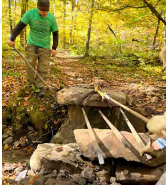
The bridge stone being placed over the two walls
