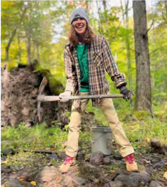
Amanda digging out drainage
