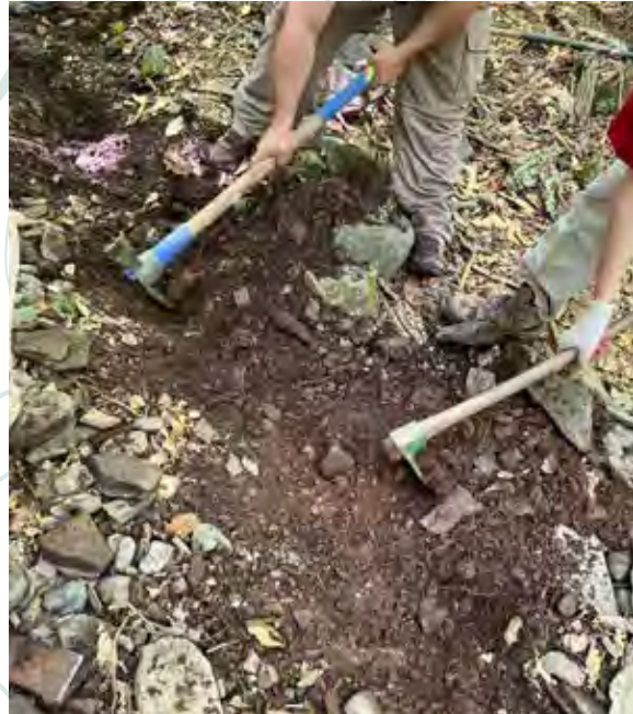
Digging another drainage path
