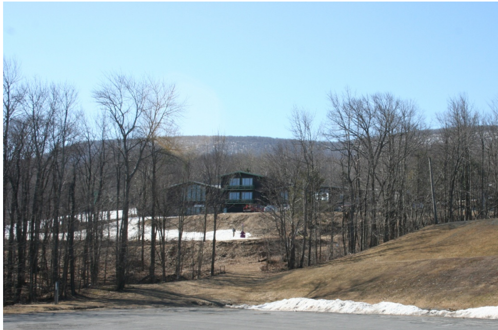
Figure 4.7-1 Existing Discovery Lodge, North Façade, from parking lots along County Route 49A (Gelli-Curci Road).
