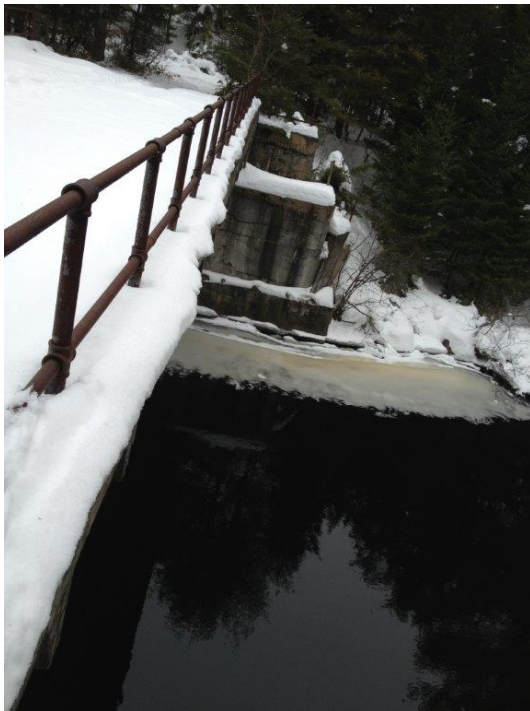
Goodman Bridge/ Concrete Bridge
