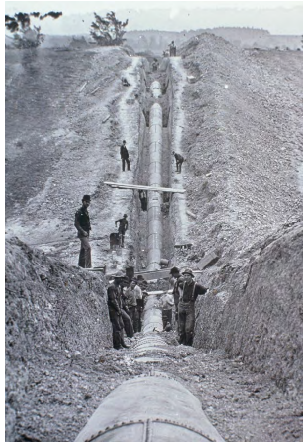
Figure 1: Water pipeline under construction between Hemlock Lake and Rochester.
