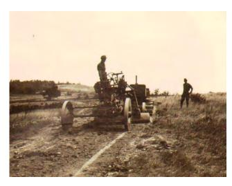
This photo was taken on July 29, 1936, of a grader being pulled by a tractor working on truck trail 202-1 by a crew out of S-123. This truck trail is still in use today, and is now the northern end of Maple Lane, and S-123 was the CCC camp located on Pine Creek Rd. Two sections of this road were relocated by the CCC, the remainder following old town road.
