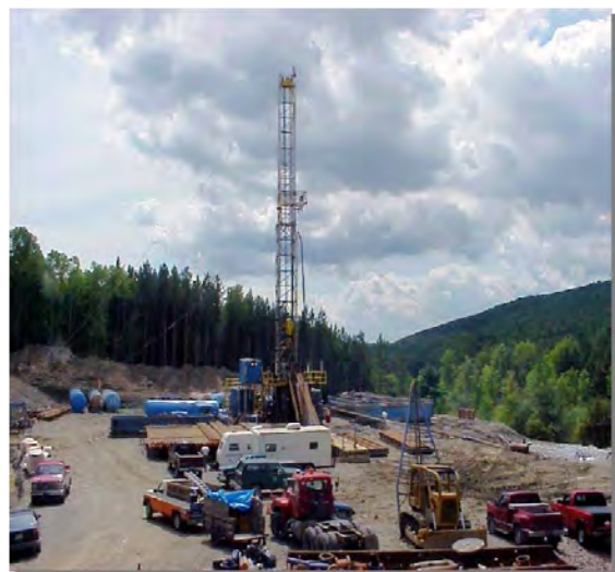
Well drilling on State Forest land over the Trenton-Black River natural gas formation
