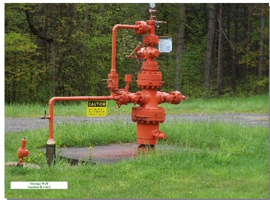
Natural gas storage well on Rock Creek State Forest in Steuben County
