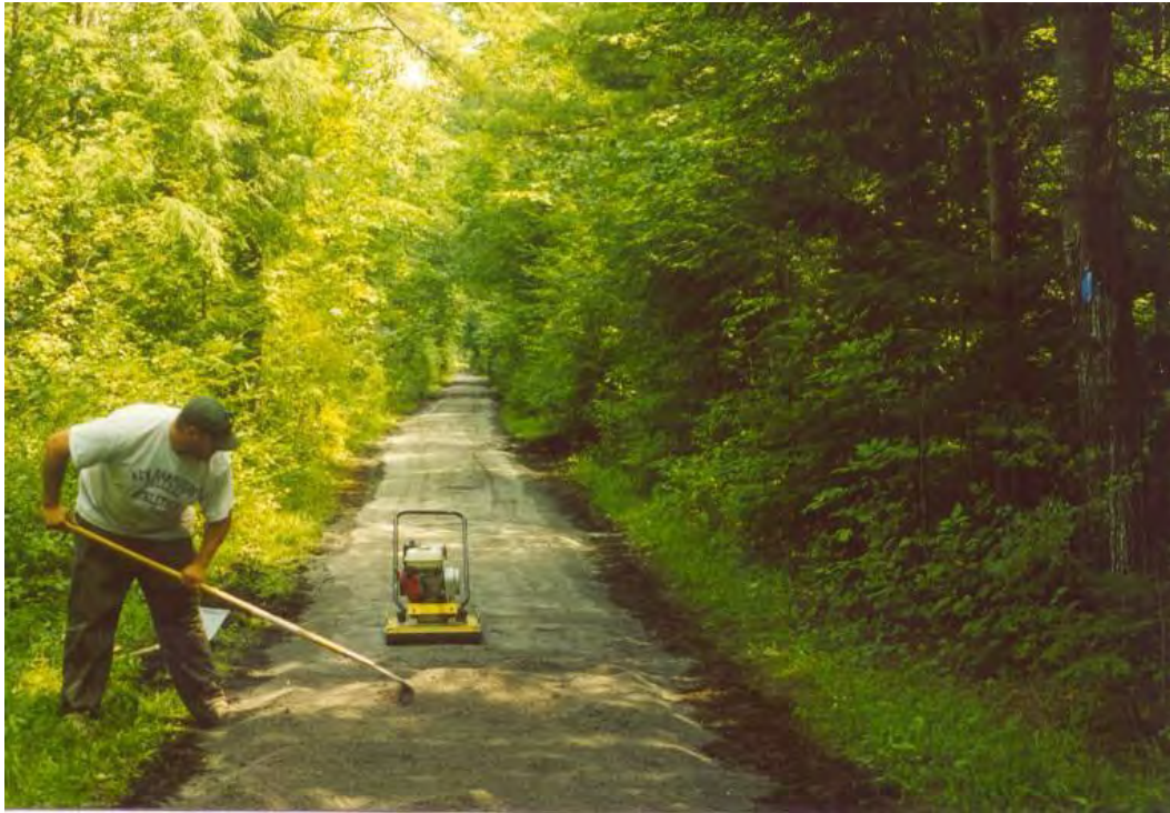
Interpretive Trail Construction at Nelson Swamp
