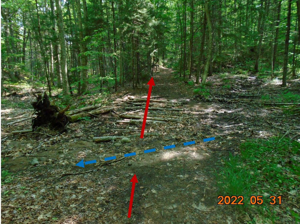
Looking East at the stream crossing. The solid red arrow delineates where the proposed turnpikes will be installed. The dashed blue arrow delineates the primary stream channel crossing the trail. Through constructing the turnpike as described (i.e., elevated from the surrounding ground and armored with rock), this stream should flow towards and cross at this single location.
