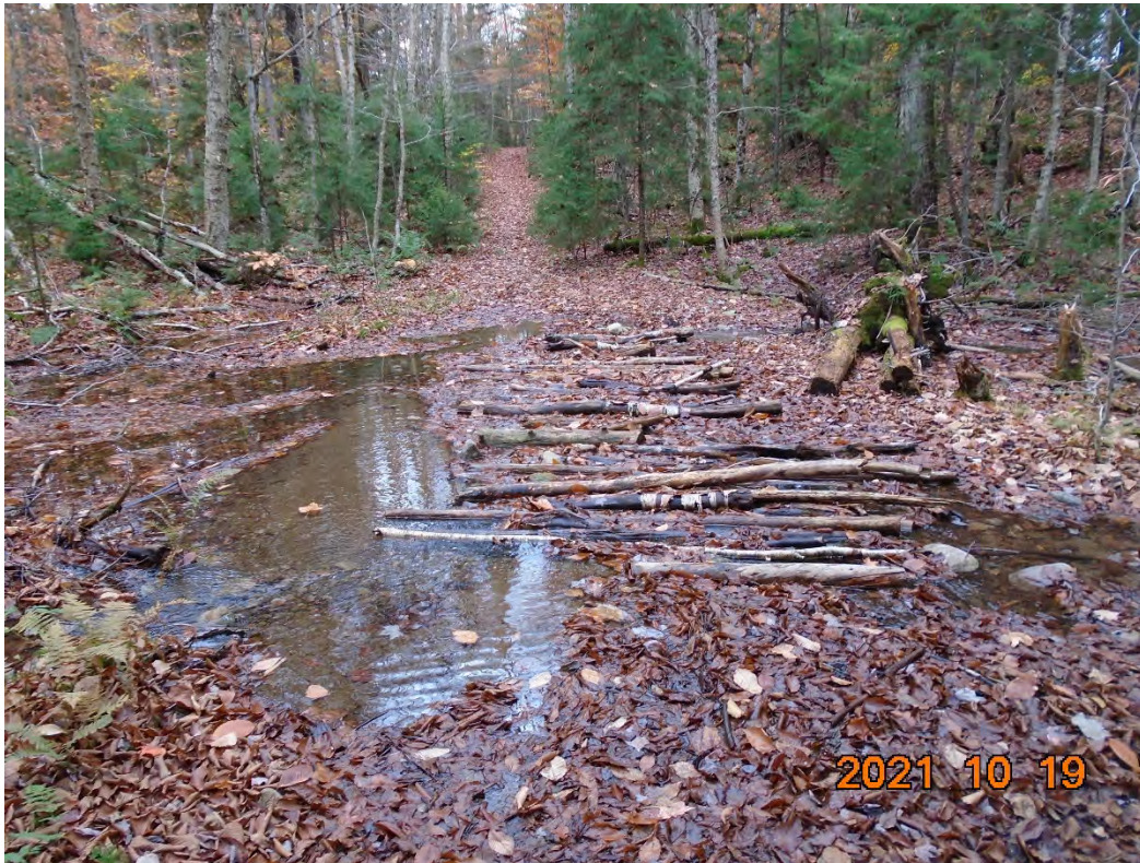
Looking West at the current stream crossing.
