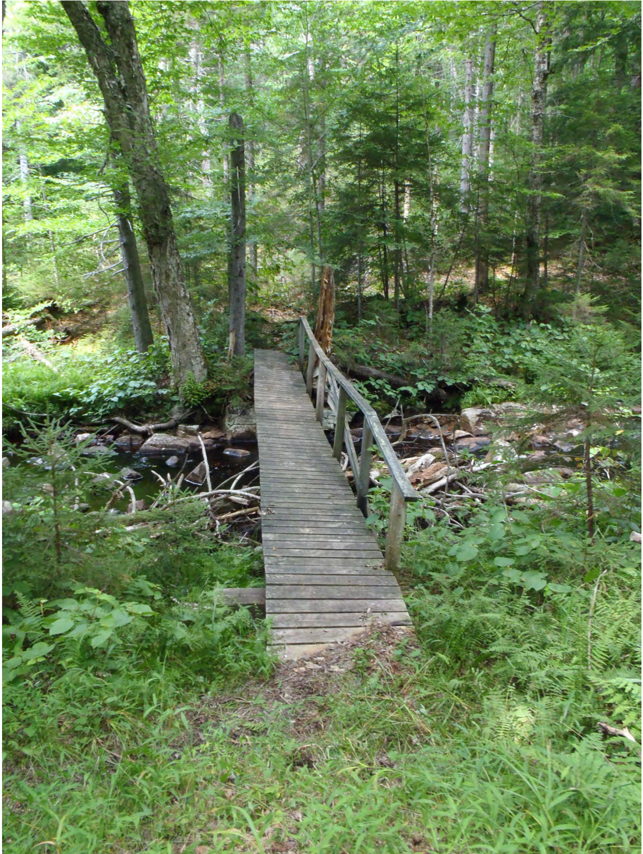
Looking North at the bridge prior to its removal
