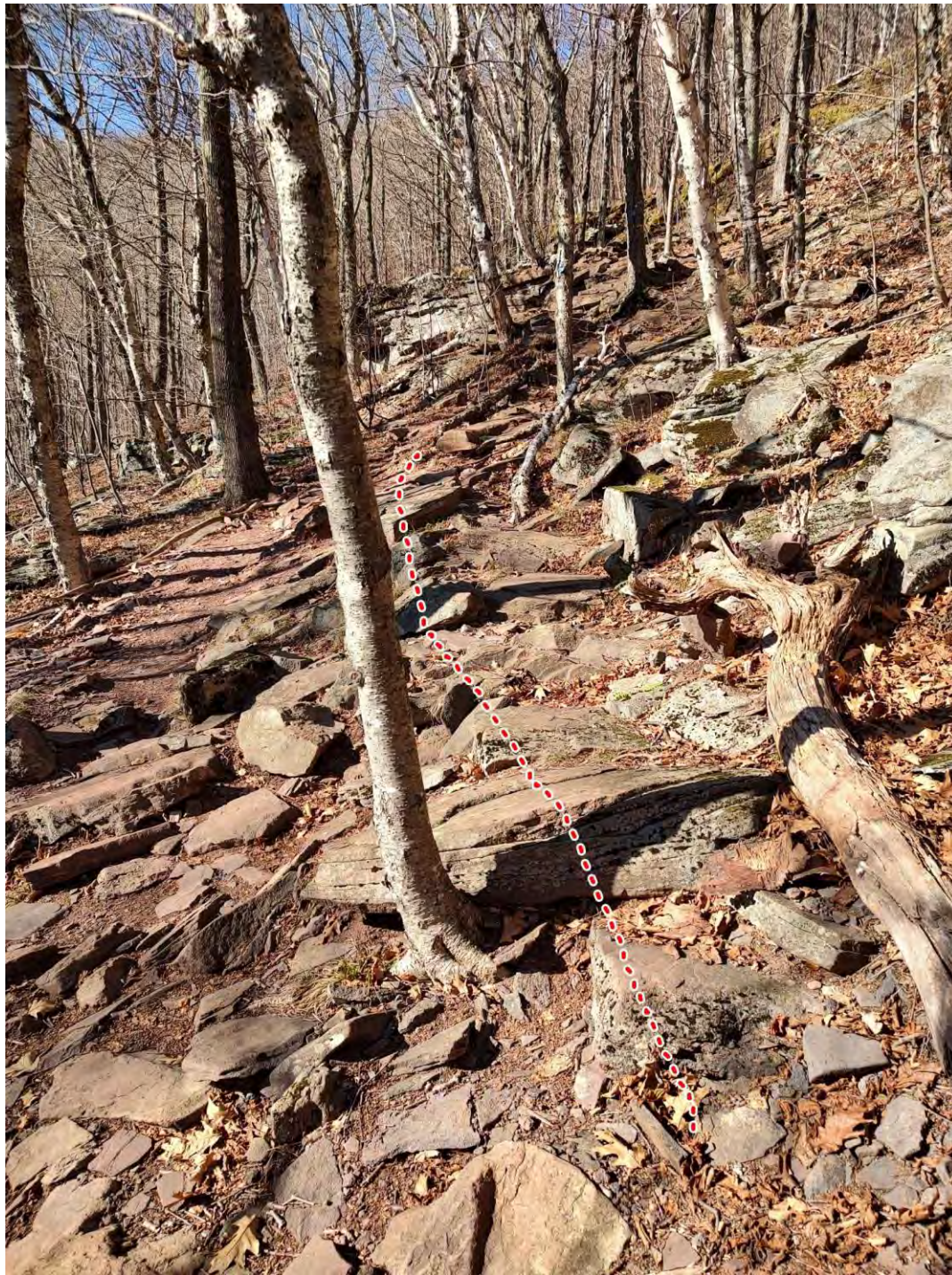
Middle staircase: Original trail alignment shown in red. Re-align staircase below birch and tighten corridor with heavy scree.
