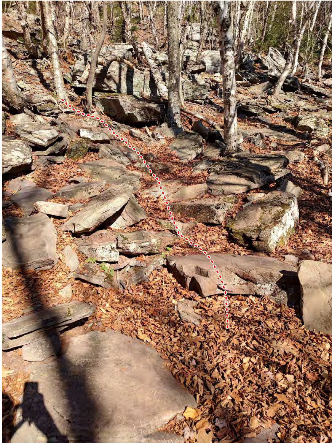
Lowermost staircase: Re-set steps. .Extend staircase below and above. Scree needs to be re-established
