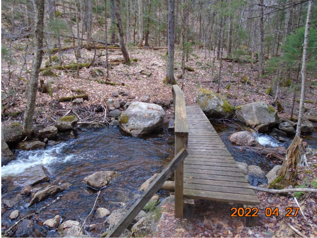
Looking west at the bridge
