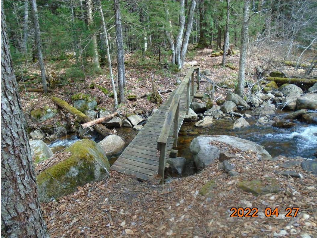
Looking east at the bridge
