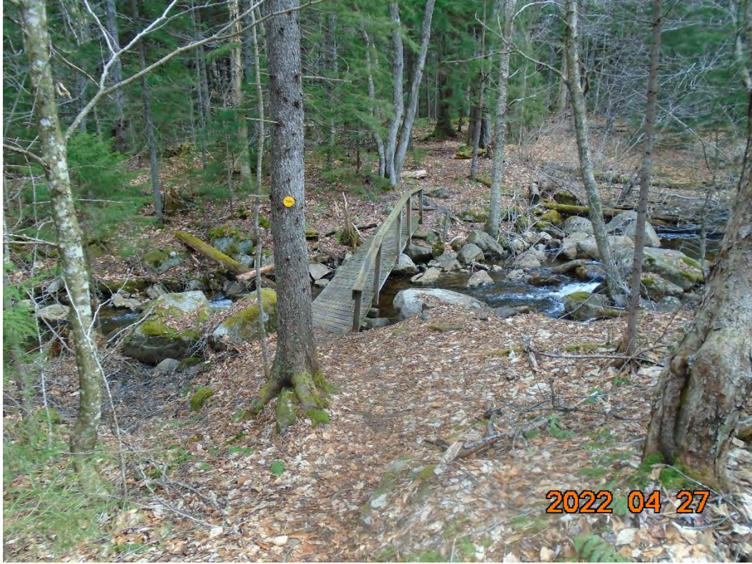
Looking east at the bridge
