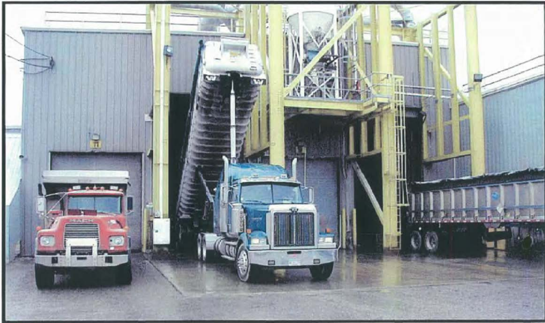
PHOTO 12 – WASTE STABILIZATION FACILITY (T04)
