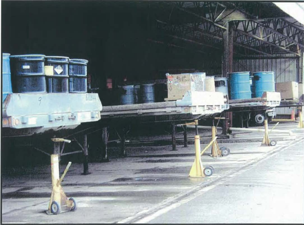
PHOTO 10 – DRUM MANAGEMENT BUILDING LOADING DOCK (S01)
