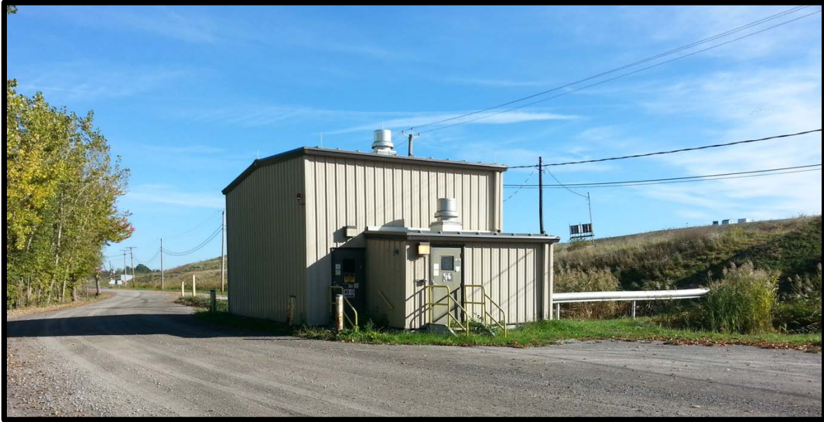
PHOTO 24 – LOCATION OF PROPOSED NEW SLF-10 HOLD TANK BUILDING LEACHATE TRANSFER RAMP (S01)
