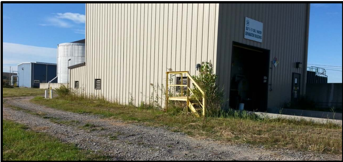
PHOTO 25 – LOCATION OF PROPOSED NEW SLF 1-11 OIL/WATER SEPARATOR BUILDING LEACHATE TRANSFER RAMP (S01)
