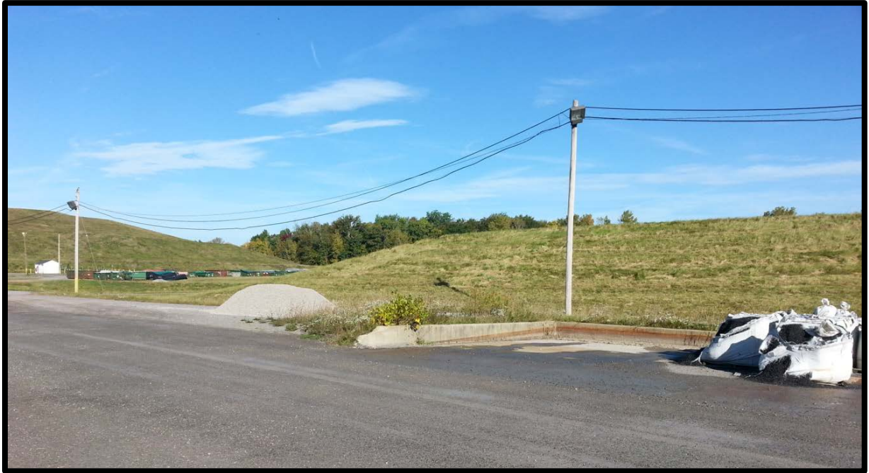
PHOTO 22 – LOCATION OF PROPOSED NEW STABILIZATION TRAILER PARKING AREA (S01)
