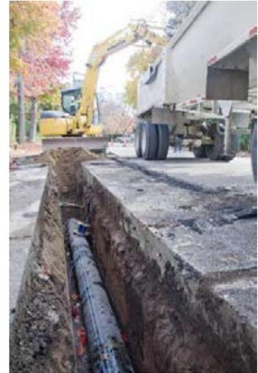
Performance Pipe manufactures pipe and fittings of high performance PE4710. Performance Pipe’s PE4710 materials are listed in PPI TR-4 with a Hydrostatic Design Stress of 1000 psi at 73°F. Where specifications and standards permit, PE4710 materials can be operated at higher pressures than PE3408 materials due to the higher Hydrostatic Design Stress rating at 73°F. PE4710 materials meet or exceed all of the requirements of the former PE3408 resin.
