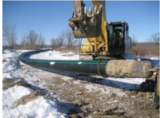
Bend radius should not be confused with the length of the pipe required to make a specific turn. Table 7 gives both the bend radius and the length required to make a 90° bend. For additional information on bending see PP407, "Small Bend Radius Big Installation Advantage" and PP819, "Field Bending of PE Pipe".
