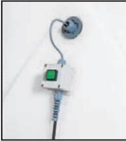
**Leak Detection Sensor**
