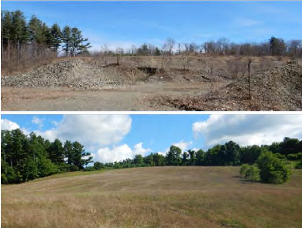
Photo 7 – Teasdale Mine – Top, site prior to grading of the mine faces. Bottom, final reclamation.
