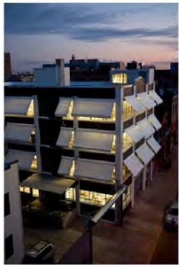
REMAINS LIGHTING FACTORY EXTERIOR II REMAINS LIGHTING FACTORY EXTERIOR III The exterior of the Remains Lighting was done in a locally sourced, green materials, and the interior lighting, and sustainable design were retained to the extent possible for their renovation and expansion work.
