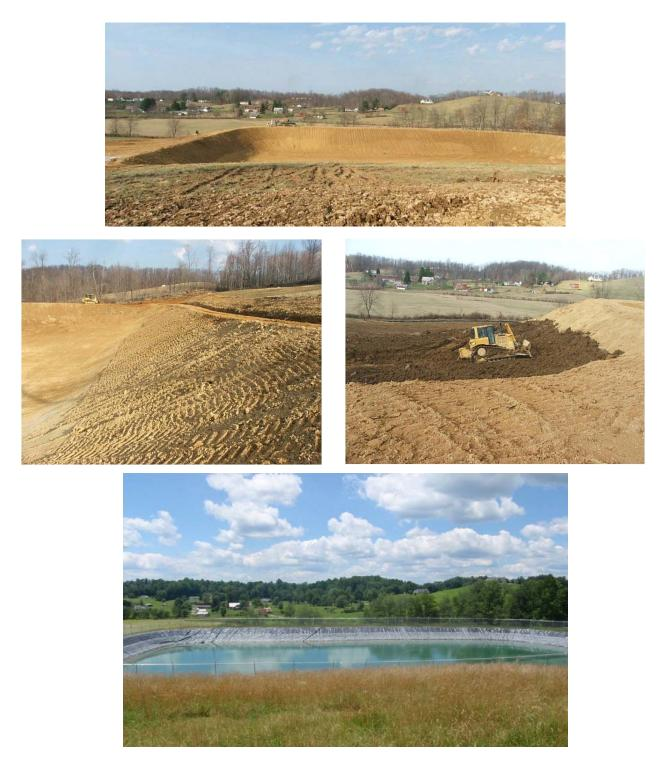
Photo 5.22 Construction of freshwater impoundment in Upshur Co. WV. Source: Chesapeake Energy
