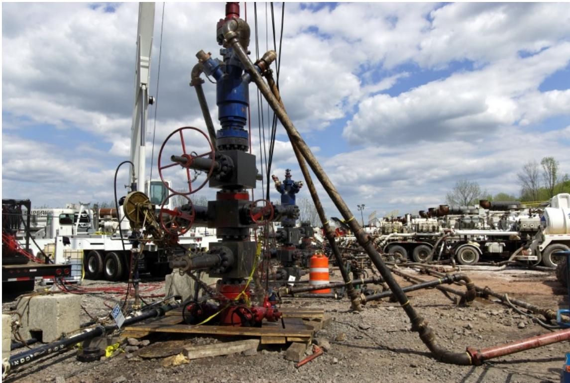
Photo 5.24- Three Fortuna Energy wells being prepared for hydraulic fracturing, with 10,000 psi well head and goat head attached to lines. Troy PA. Source: New York State Department of Environmental Conservation 2009
