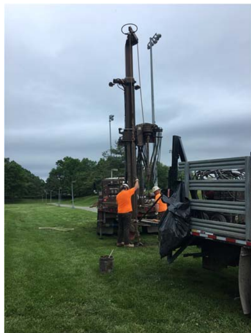
Photo 2.4: Monitoring well installation at an inactive landfill.
