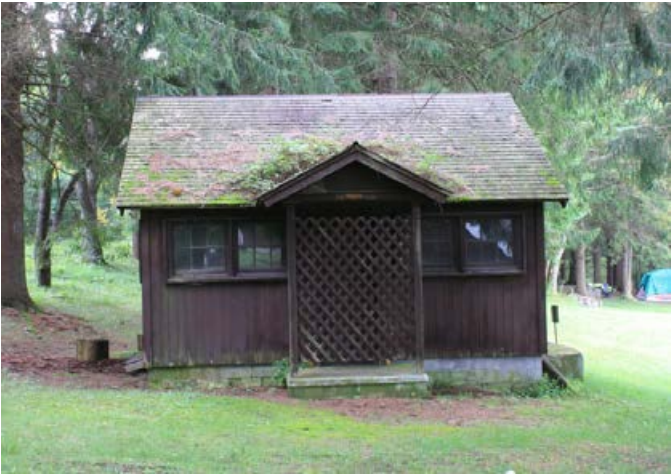
Figure 7 Storage Bldg (Old Pit Toilet)
