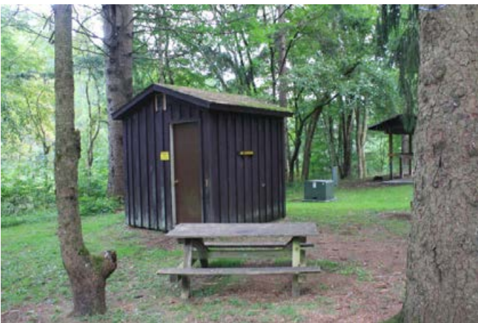
Figure 11 Spruce Grove UV Filtration Bldg
