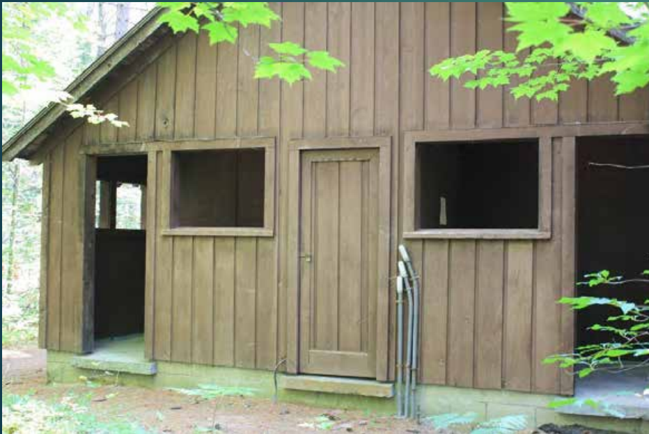
Comfort Station #3 –Slop Sink Entrance
