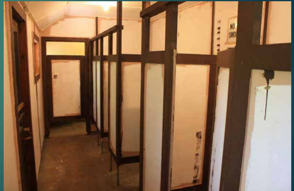
Comfort Station Interior
