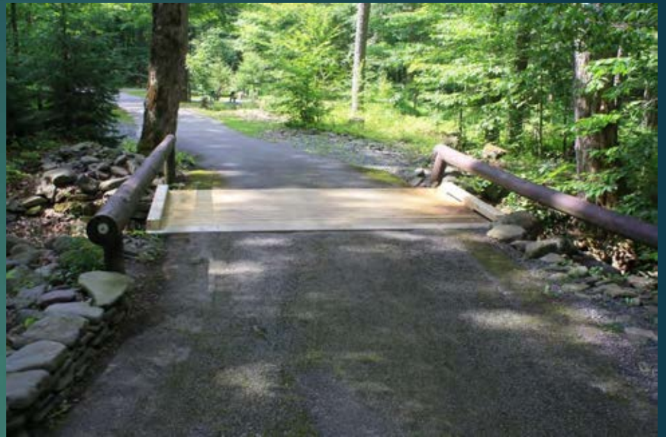
Bridge Near Site 17
