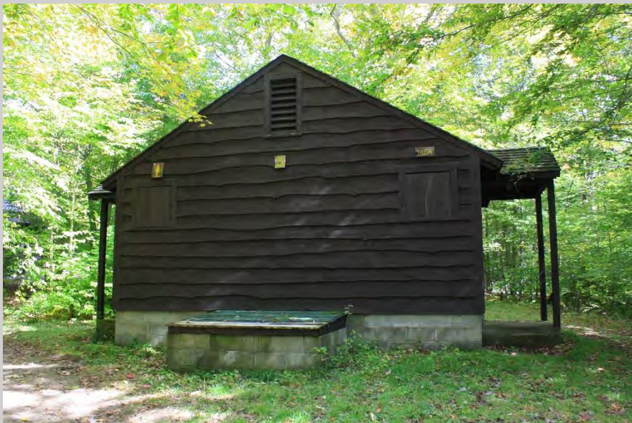
Comfort Station # 3 (Vault)
