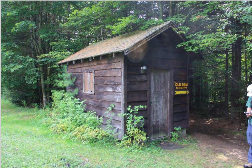
Sewage Chlorinator Building (not in use)
