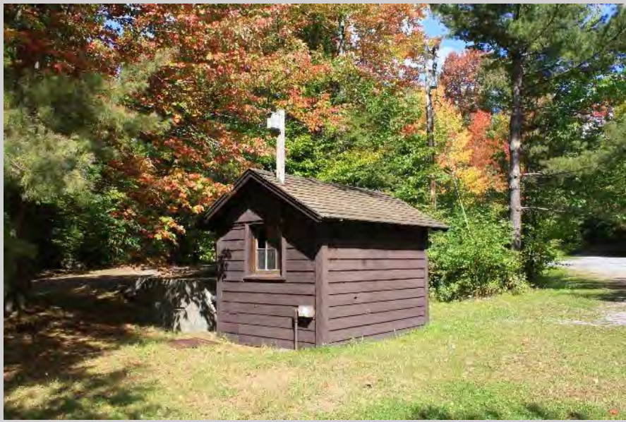
Limekiln Lake Chlorination Bldg
