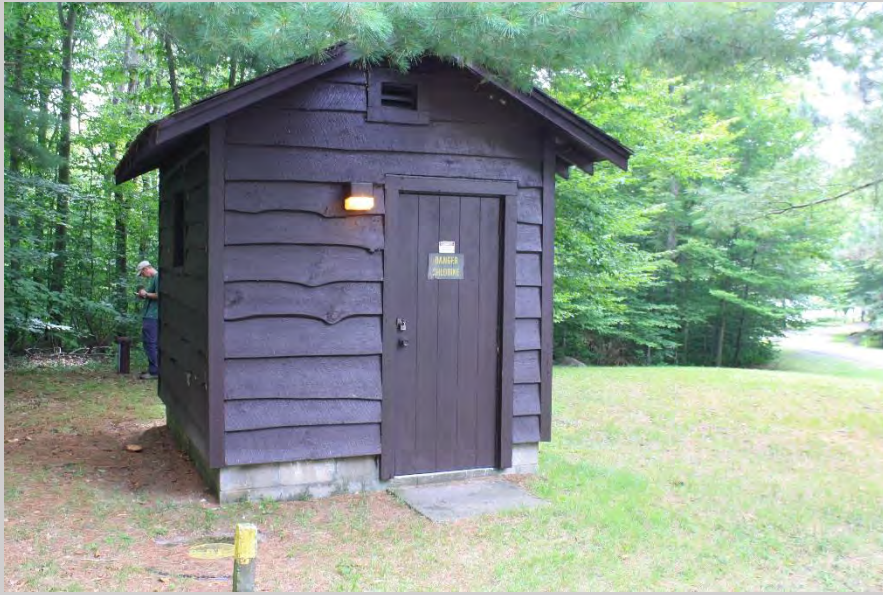
Pump House and Chlorinator
