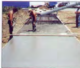
The deck concrete is poured, vibrated, and screeded.
