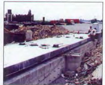
The load cells are installed, and the deck is raised 6 inches.
