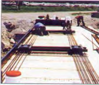
Deck assembly begins with side channels, steel nests and rebar.
