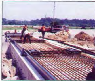
A double layer of rebar is completed.
