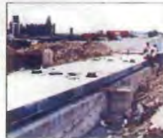
The load cells are installed, and the deck is raised 6 inches.
