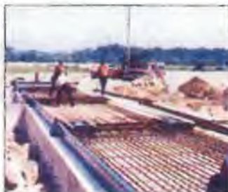
A double layer of rebar is completed.
