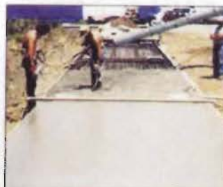
The deck concrete is poured, vibrated, and screeded.
