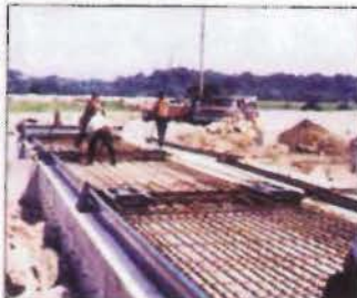
A double layer of rebar is completed.
