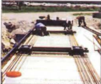
Deck assembly begins with side channels, steel nests and rebar.
