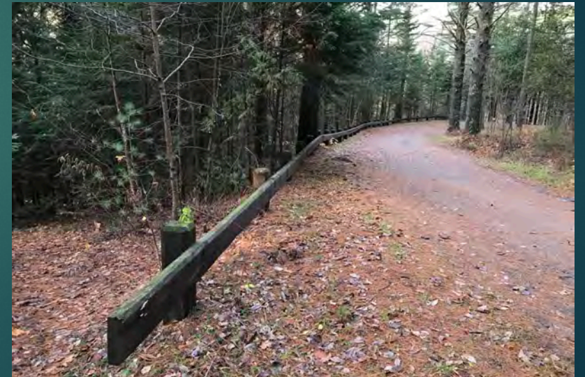
Paved Road with Guardrail into Camping Area.
