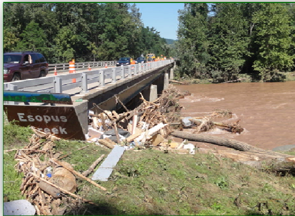
Woody debris blocking bridge openings should be removed.
