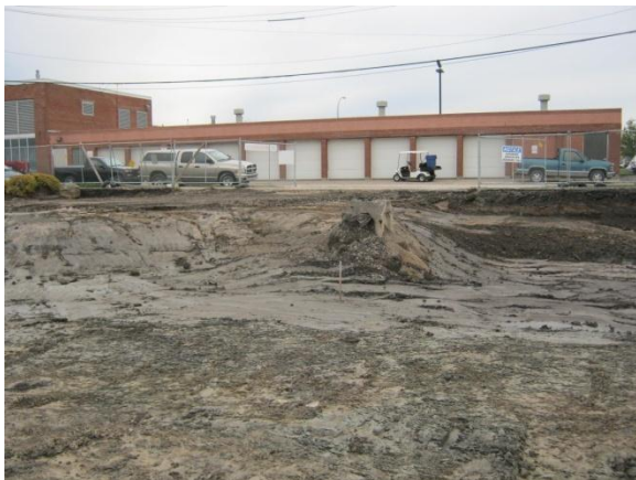
Photo 15 – Phase 4 – Excavated to Clean Soils
