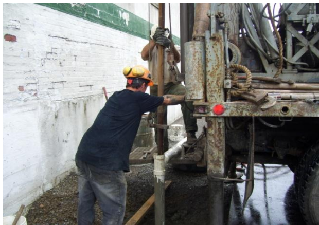
Photo 3 – Monitoring Well Installation
