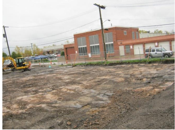
Photo 10 – Phase 1b – Excavated to Clean Soils
