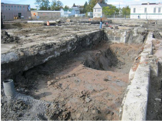
Photo 7 – UST #1 & 2 Tank Pit – After Removal
