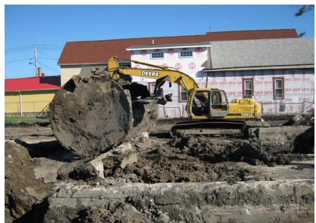
Photo 6 – UST Removal – Phase 3b
