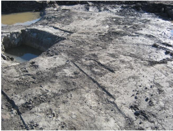
Photo 13 – Phase 3a - Excavated to Clean Soils
