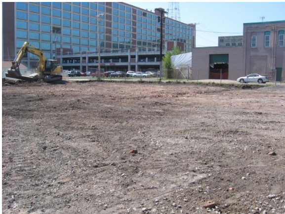
Photo 9 – Phase 1a – Excavated to Clean Soils
