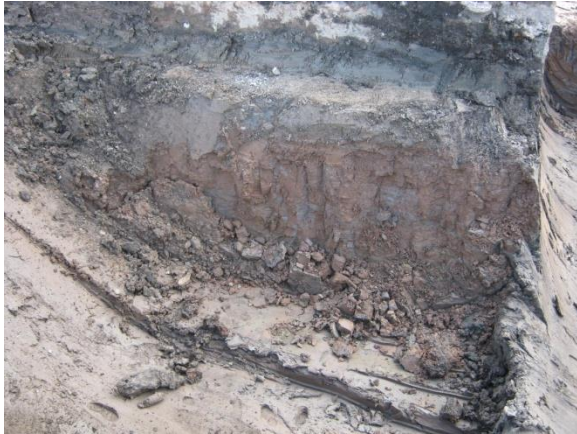
Photo 8 – UST #3 Tank Pit – After Removal
