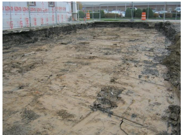
Photo 12 – Phase 2b – Excavated to Clean Soils
