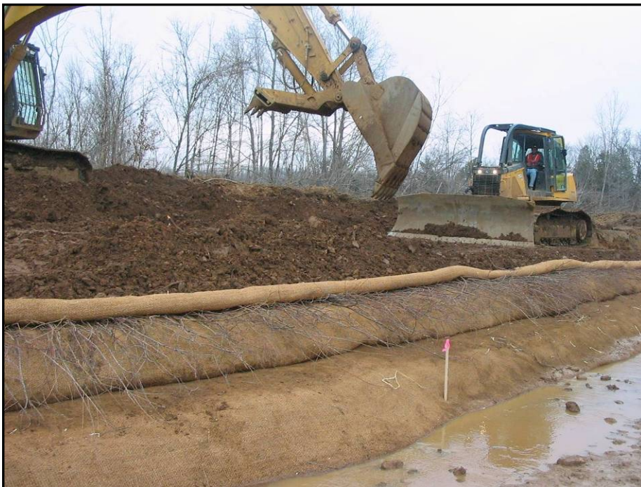
Wrapped earth with branch packing during installation.
