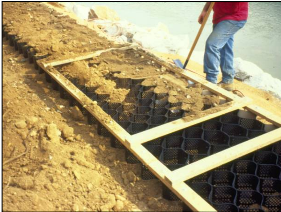
Geocells during installation.
