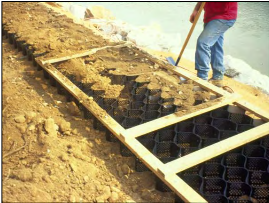
Geocells during installation.
