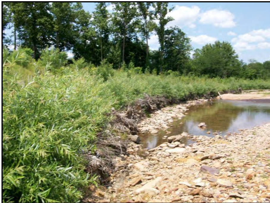
Rootwads with branch packing and live stakes after one year.
