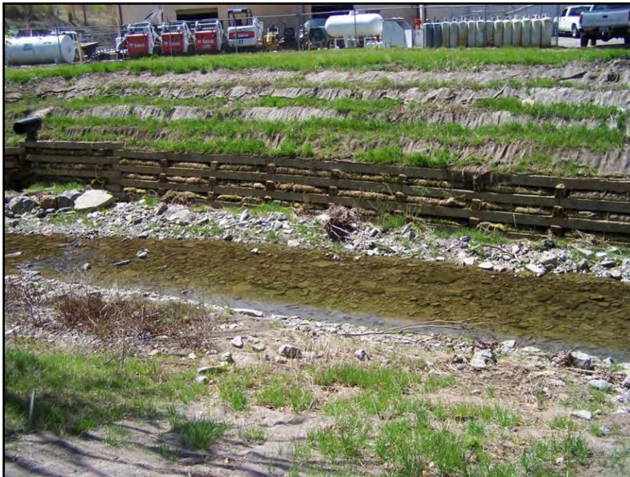
Crib wall with wrapped earth.
