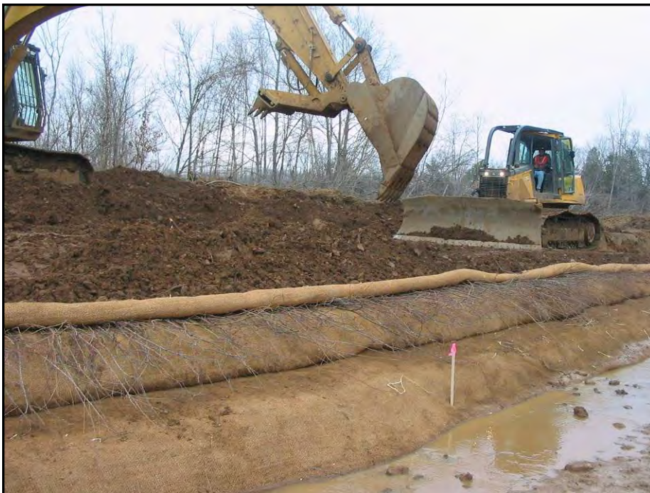
Wrapped earth with branch packing during installation.
