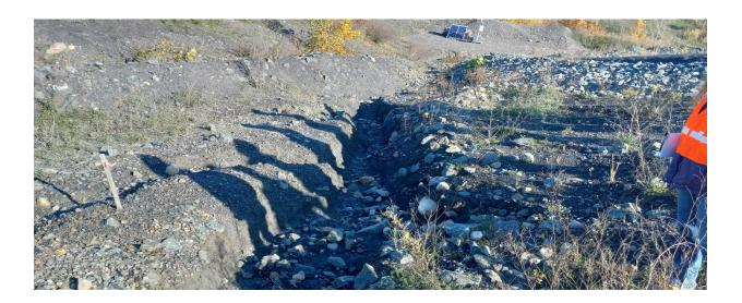
The photographs below document the poor quality of stormwater discharge from the SOSA into the Quarry Pond. Such conditions do not comply with the terms of the SWPPP.
